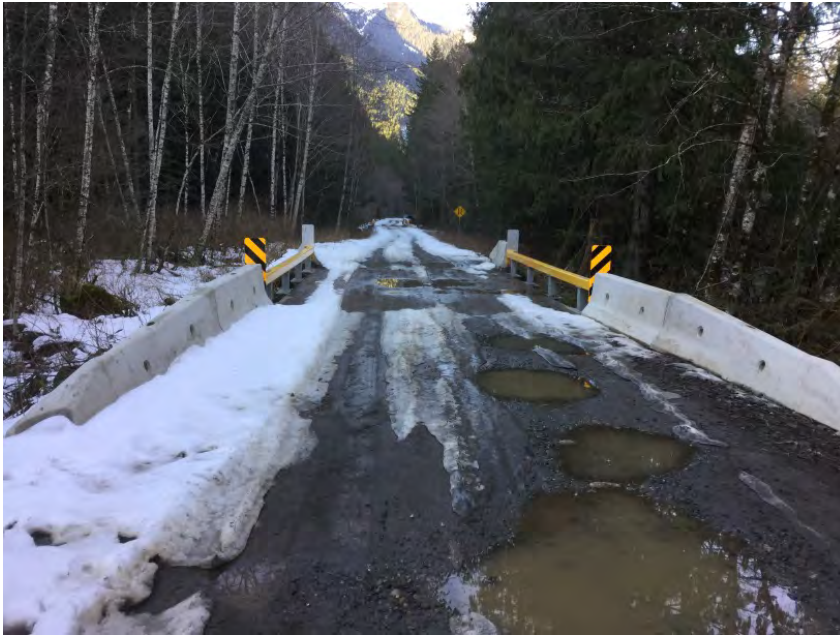
Approach from Right Bank when facing downstream
