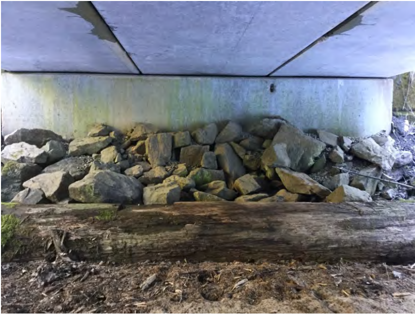
Right Bank Abutment when facing downstream
