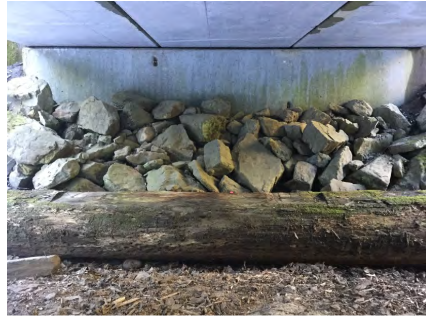
Left Bank Abutment when facing downstream
